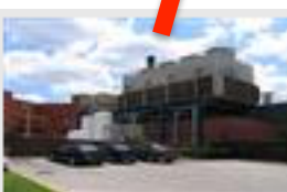
Medical Center Heating and Cooling Plant [0085]
