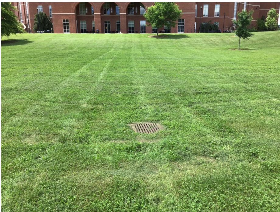
Sink hole in Southern Basin from surface.
