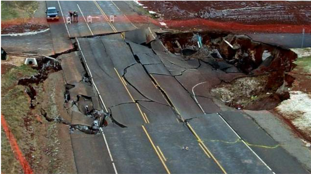
Western Kentucky University Department of Geography & Geology A sinkhole collapse in February 2002 undermined part of Dishman Lane in Bowling Green, creating an opening approximately 150 feet wide and 20 feet deep in the three-lane road. Repairs cost about $1 million, according to published reports. No one was injured, but several vehicles were trapped, with at least two falling into the opening.
