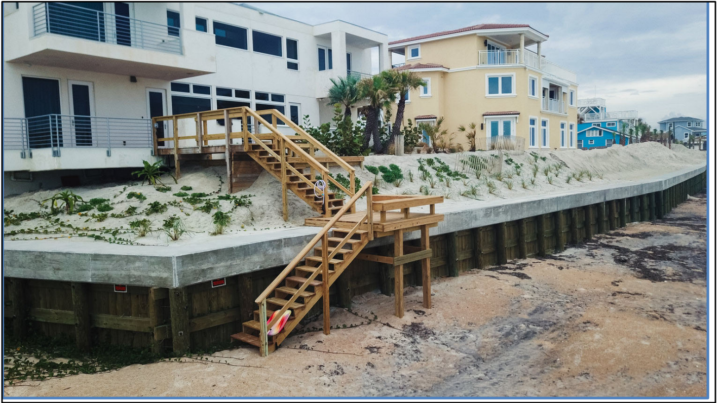
Hardening of the shore through sea walls
