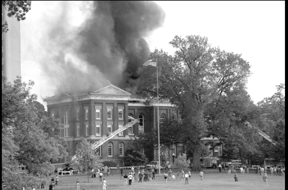
Administration Building May 15, 2001
