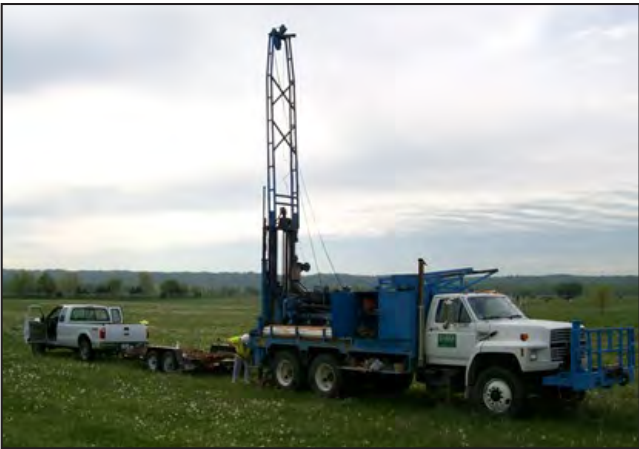
Figure 12. Installation of a USGS groundwater-monitoring well near West Point, Ky.
