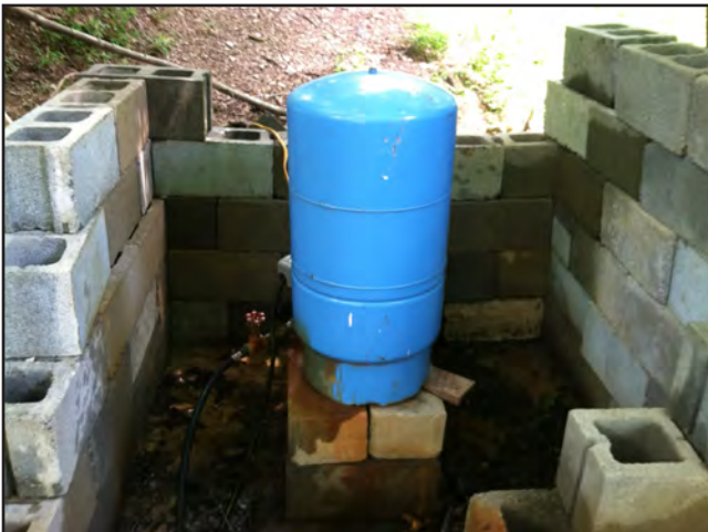
Figure 19. Pressure tank for a water well (located behind the tank), which was investigated because the owner thought the well's high iron content may have been caused by local coal mining.
